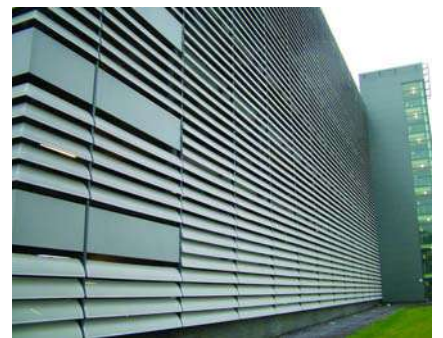
Addenbrookes Hospital, Cambridge. Perforated cladding and perforated Solarfin for screening and ventilation.
