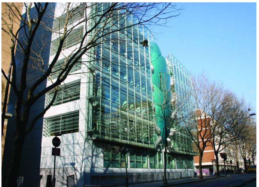
Arup Fitzrovia, London. Fixed Solarfin supported by drop rods, and Universal Louvre fitted to plant rooms.
