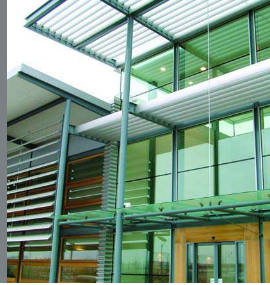
John Lewis, Cambridge. Solarfin fitted both to the customer entrance canopy and in front of the facade.
