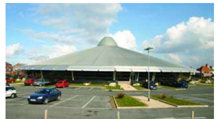
Crosby Leisure Centre, Liverpool. Stucco embossed aluminium louvres set onto prefabricated faceted structure.
