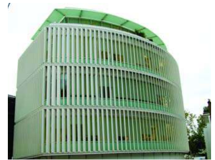
Clear Channel Outdoor, London. Both fixed and movable vertical Solarfin louvres installed onto the facade.
