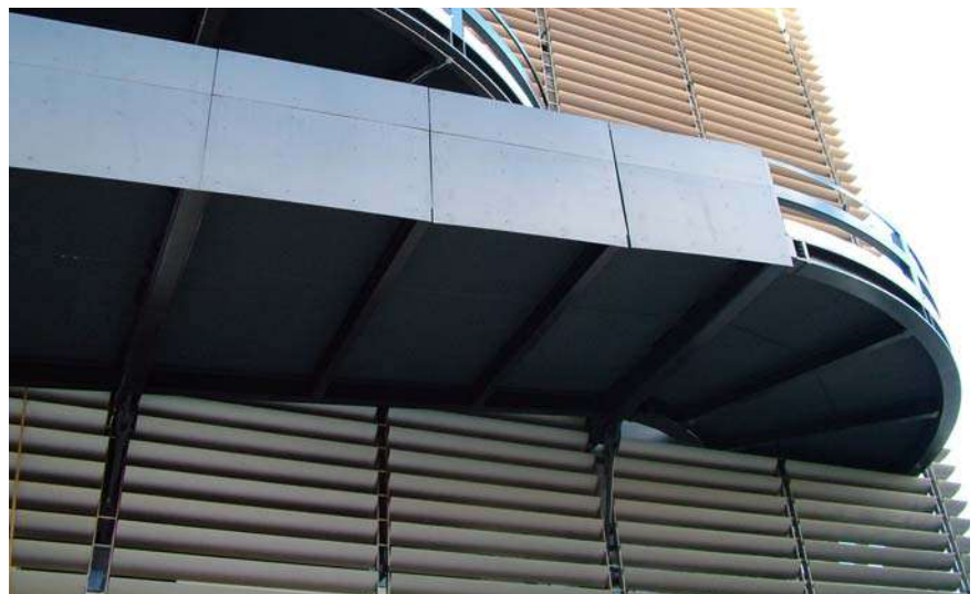
Paradise St Car Park, Liverpool Fixed Solarfin with special ladder mullion system and mitred corners.
