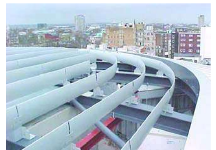
Aldersgate, London. Curved horizontal screening fins and panelised louvre panels.
