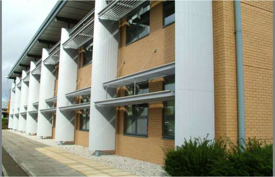
Truckstop, Dunstable. Bespoke vertical fins and Solar C.
