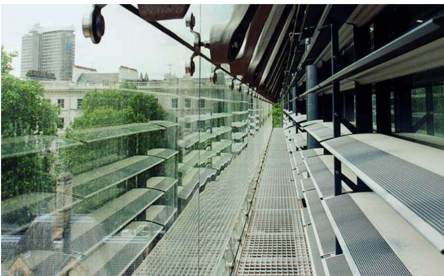
Natural History Museum, London. Between the Colt glass façade and walkway of the stunning South façade is a bespoke, controllable fin, which is half perforated to provide additional daylight when in the closed position
